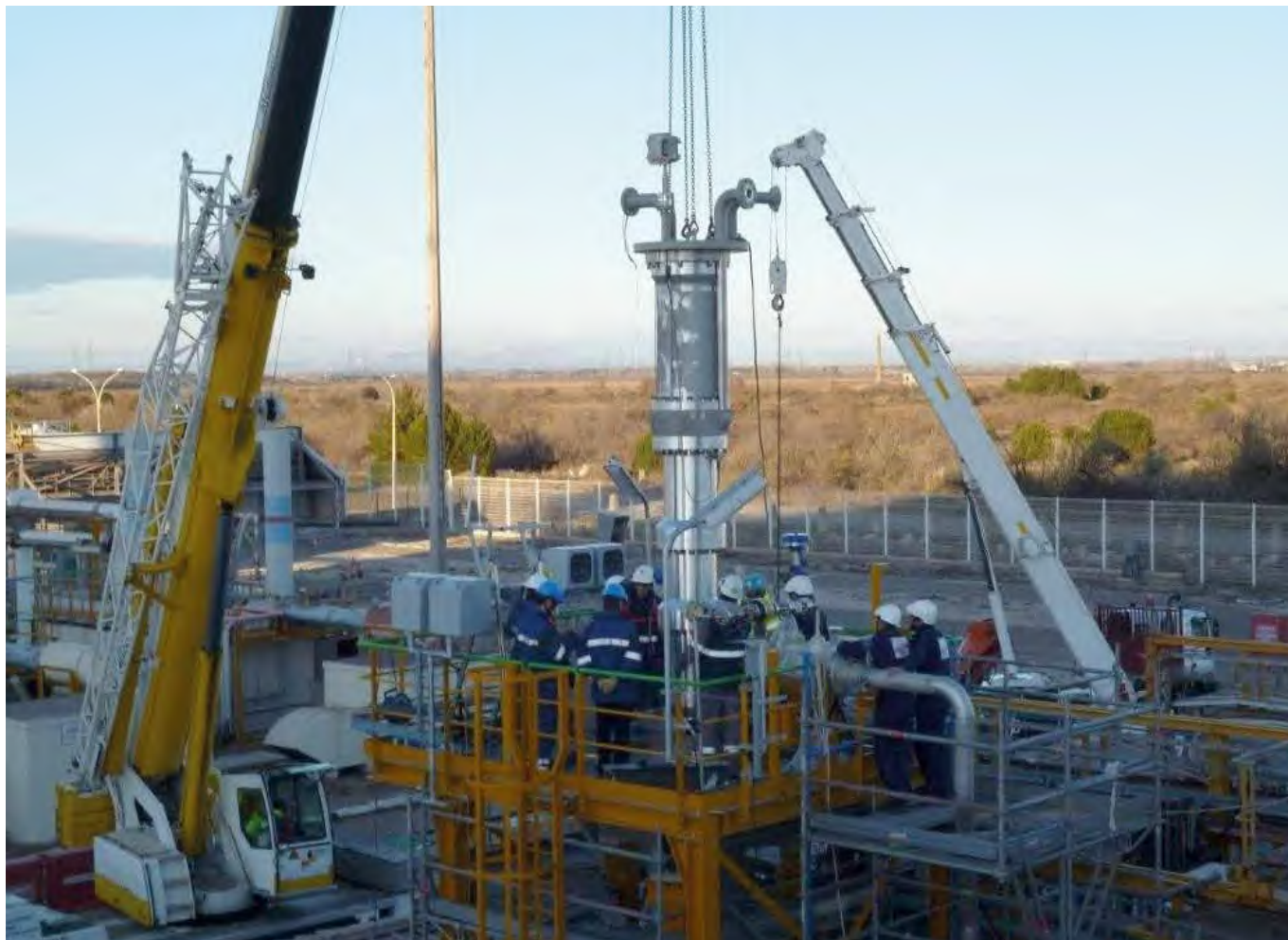
▲ Geveke helps to install a Nikkiso cryogenic centrifugal pump
